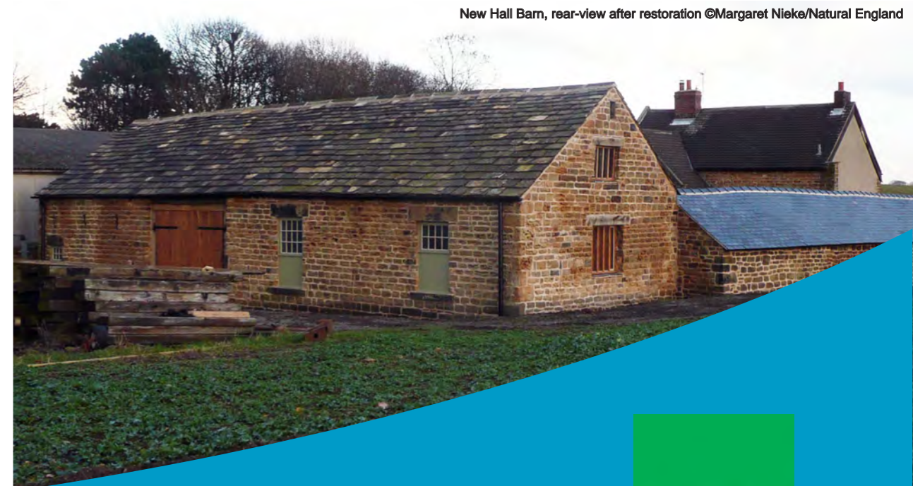
New Hall Barn, rear-view after restoration ©Margaret Nieke/Natural England
